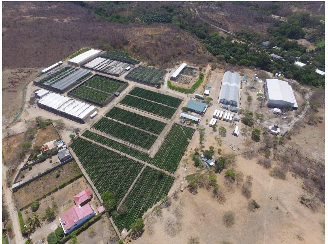
Figure 9: Facility in Colombia
