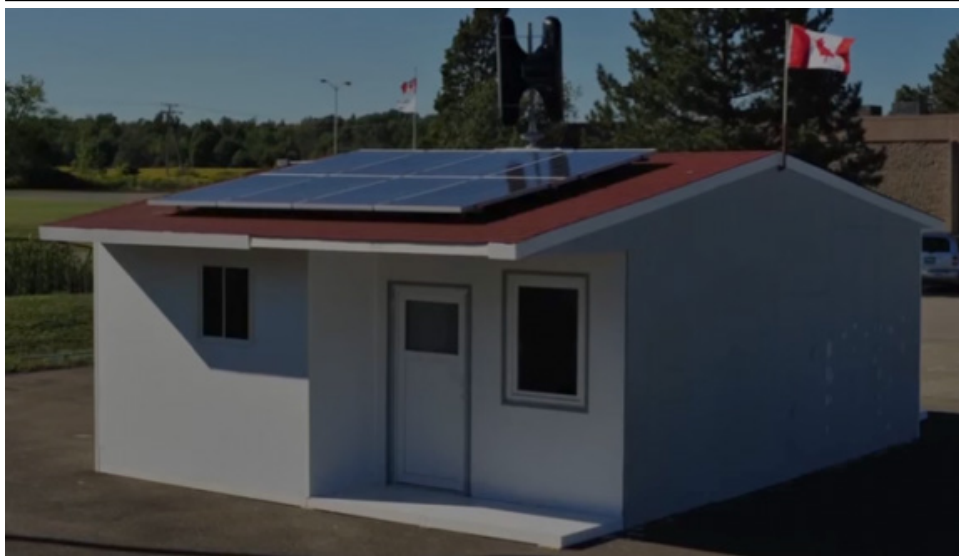
Figure 4. EHT's Advanced Modular Housing System with solar panels
